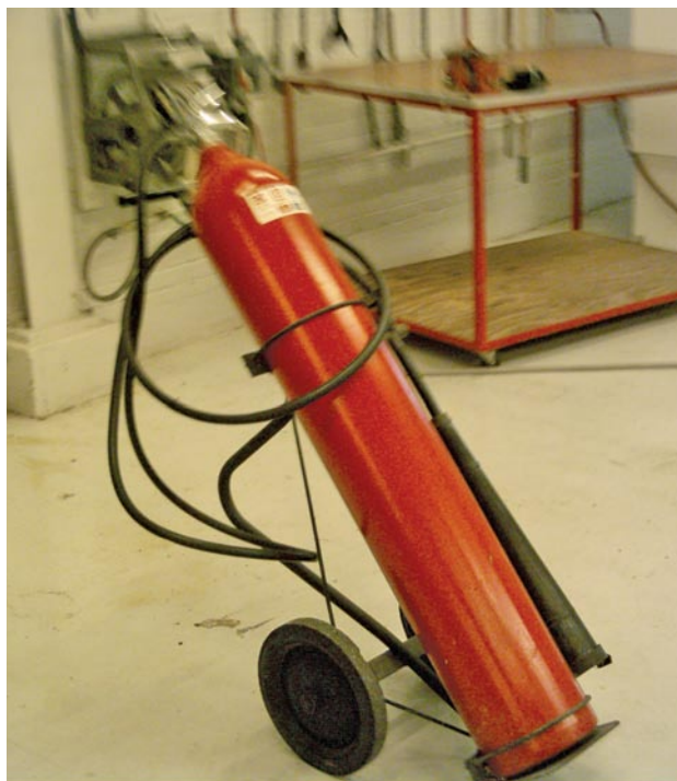
Figure 11-4. Carbon dioxide fire extinguisher.
